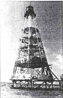
Alligator Reef Lighthouse being painted recently. Photo by Jerry Biggs.
