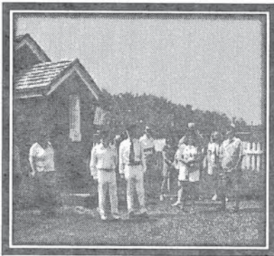
Keepers and visitors at Ponce Inlet Lighthouse
