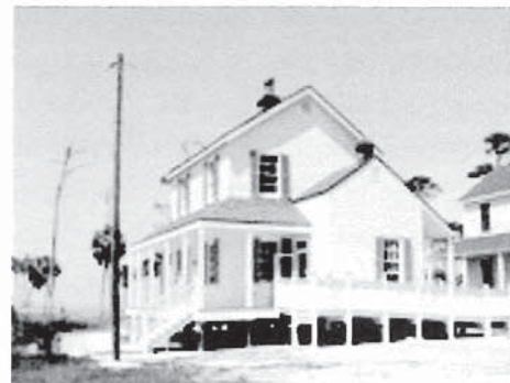
Before and after restoration of "Sleeping Beauty," one of the original keeper's houses at Cape San Blas Lighthouse
