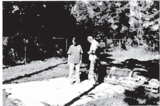
Above, Ken and Joan are at the foundation/concrete pad that the City of Carrabelle has donated to the Crooked River Lighthouse. The historic Wash House will be moved to this location.
